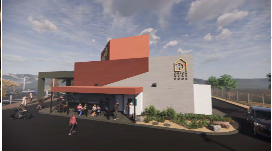
VIEW WEST FACADE / RESTAURANT SEATING FROM PARKING LOT
